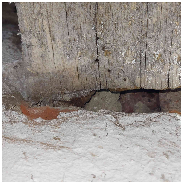
Obr. 16: ST 1, degradace trámovkou detail
